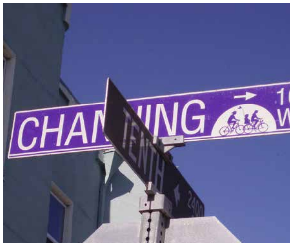
Custom street signs can also act as a type of confirmation sign, to let all users know the street is prioritized for bicyclists.
