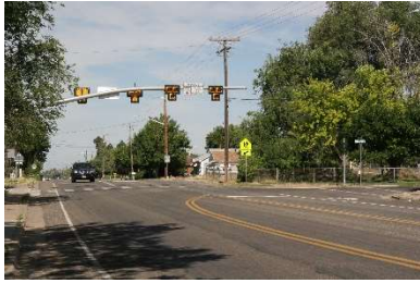
Figure 7: HAWK Crossing in Clearfield
