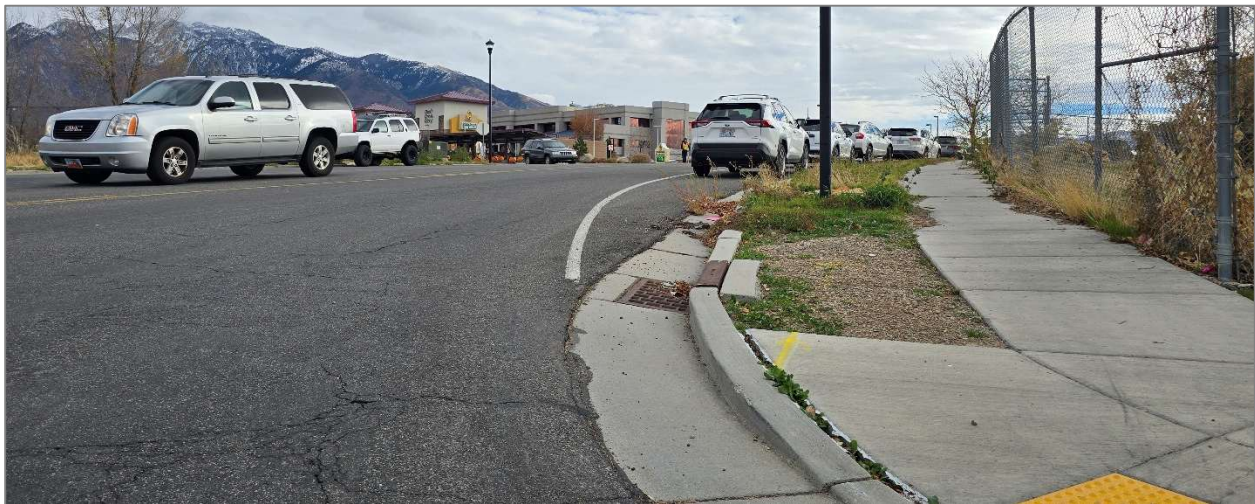
Figure 15: Sight lines for eastbound left-turning vehicles are constrained
